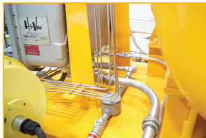
CONDUIT ISOLATED WIRING
